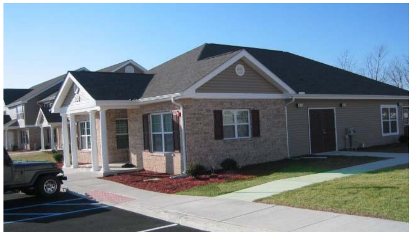
Old Landing I and II is a community of apartments and townhouses, produced by Millsboro Housing for Progress. A unique feature of Old Landing II is a special subsidy reserve which supports six of the units, allowing them to serve families earning no more than 30% of area median income. This rental assistance was provided by DSHA through the Housing Development Fund.
