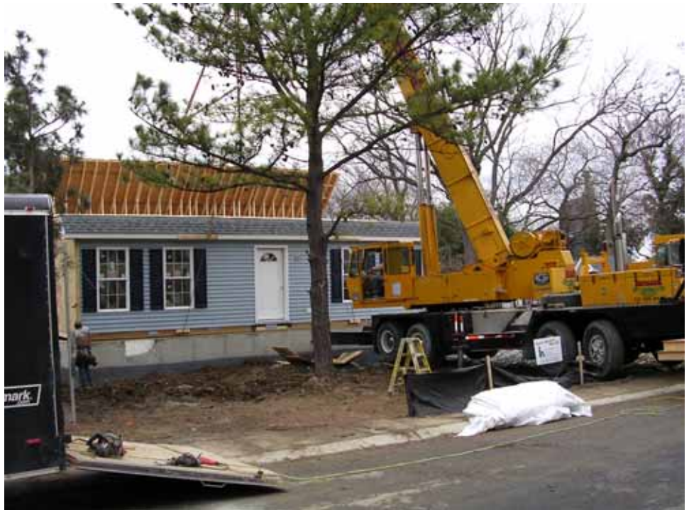
In-fill development in Belvedere by Interfaith Community Housing Delaware, making use of modular housing component.
